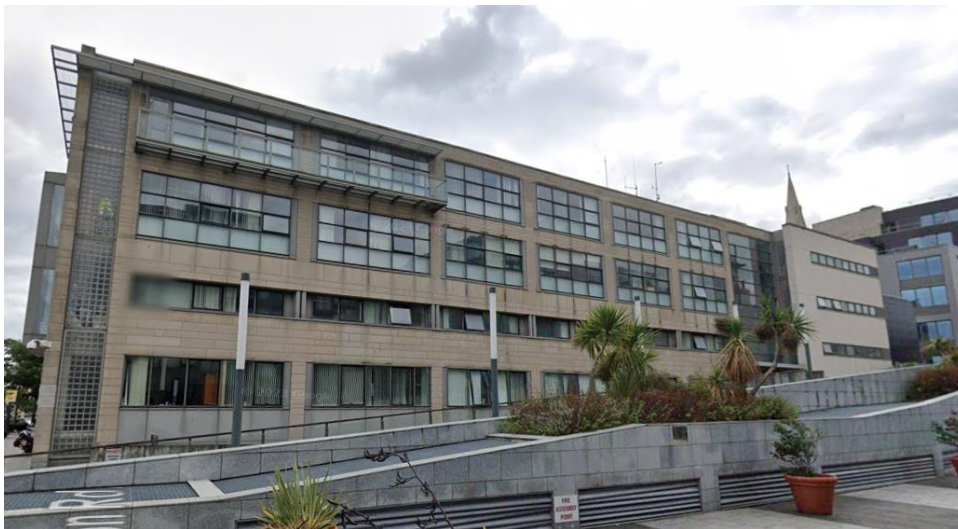
Figure 5: County Hall – BIPV Solar Panels
