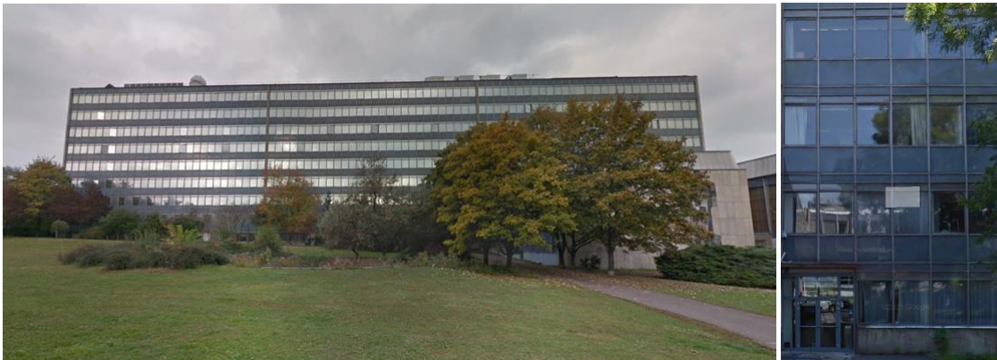
Figure 38: South façade of Building B
