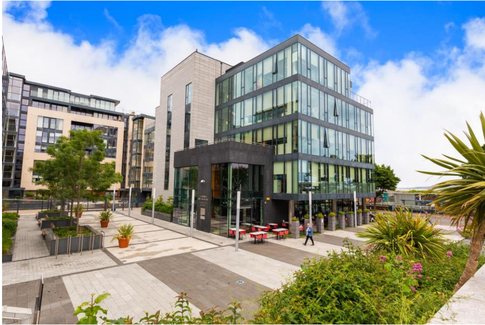
Figure 9: Harbour Square – Integration of BMS to Digital Twin
